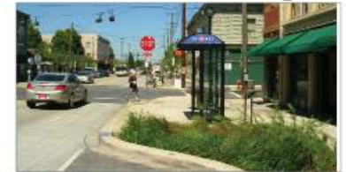
Green infrastructure can create a safer and more pleasant environment for bus riders and pedestrians.
