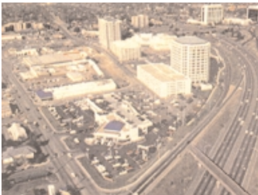
Figure 8- Existing conditions at Colorado Blvd. and Evans Avenue (looking N.W. from I-25 and Evans Avenue)
