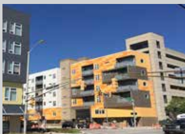
Mosaic Development (Indianapolis) After wrap - elevation view
