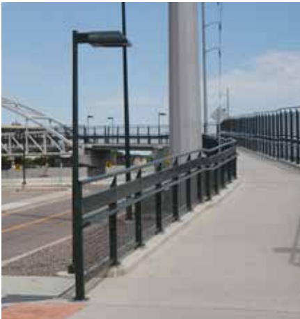
Pedestrian Bridge at Colorado Station
