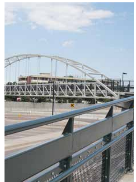
Existing Pedestrian Bridge at Colorado Station
