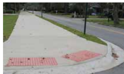
A complete network of curb ramps and sidewalks enhance the pedestrian environment
