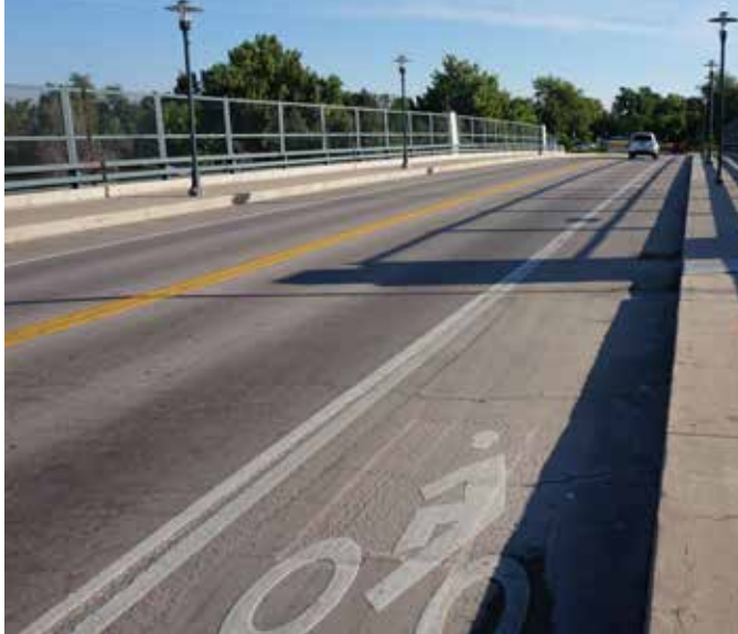
Existing bike lane at Franklin St.
