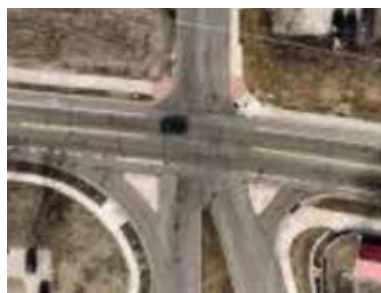
Existing Intersection at Buchtel Blvd. and Monroe St.
