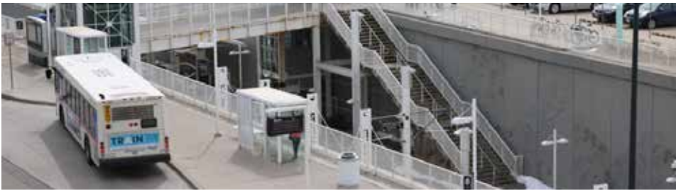
Bus Station at Colorado Station with Light Rail Station below grade
