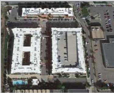
The District - Parking structure wrap in Denver
