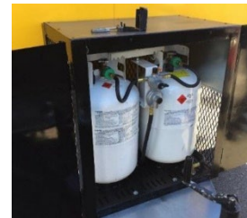
Propane Tanks with Dual Regulator
